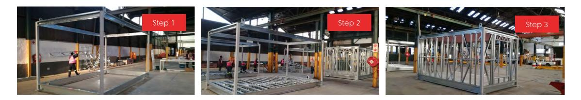
6mm/4mm/3mm + 0.8mm - 1mm Lightweight Steel Structure (LGS)
